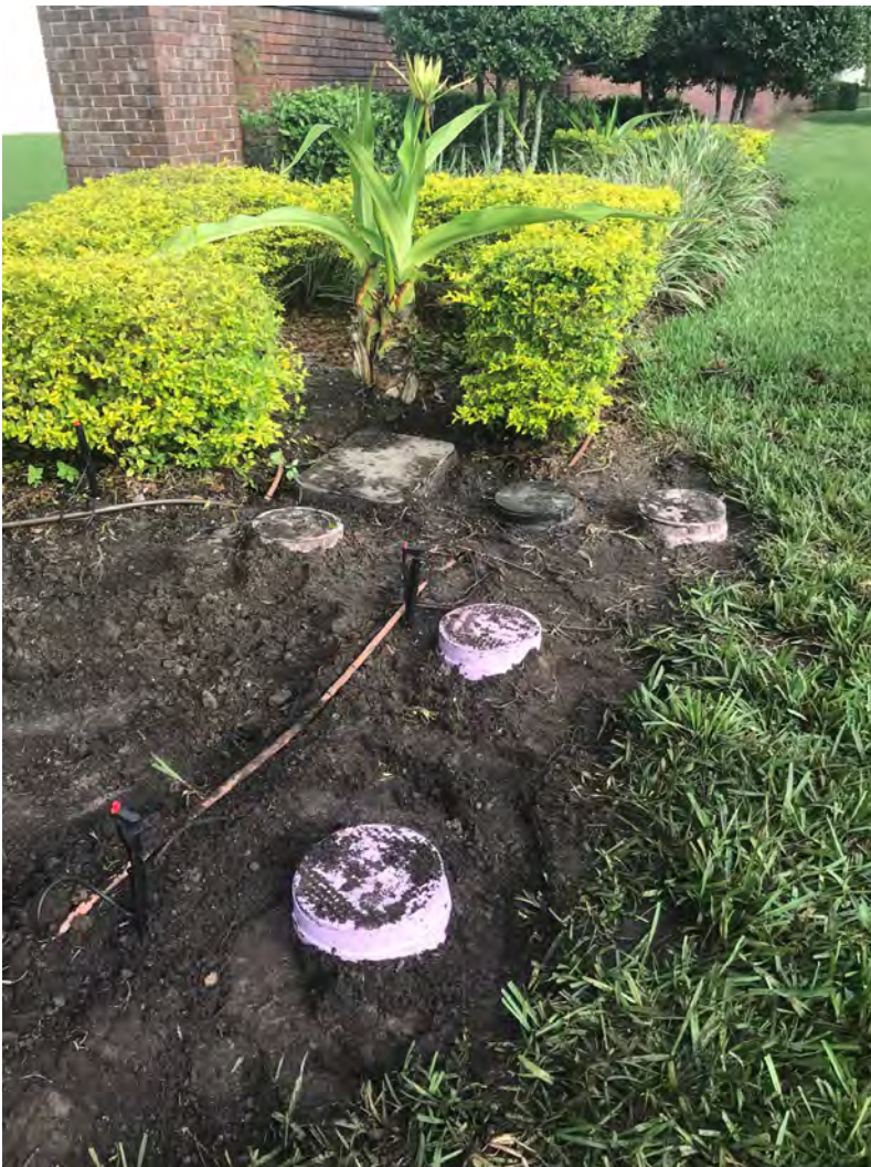
Exposed irrigation valves at Pleasant Plains and Lagerfeld.
