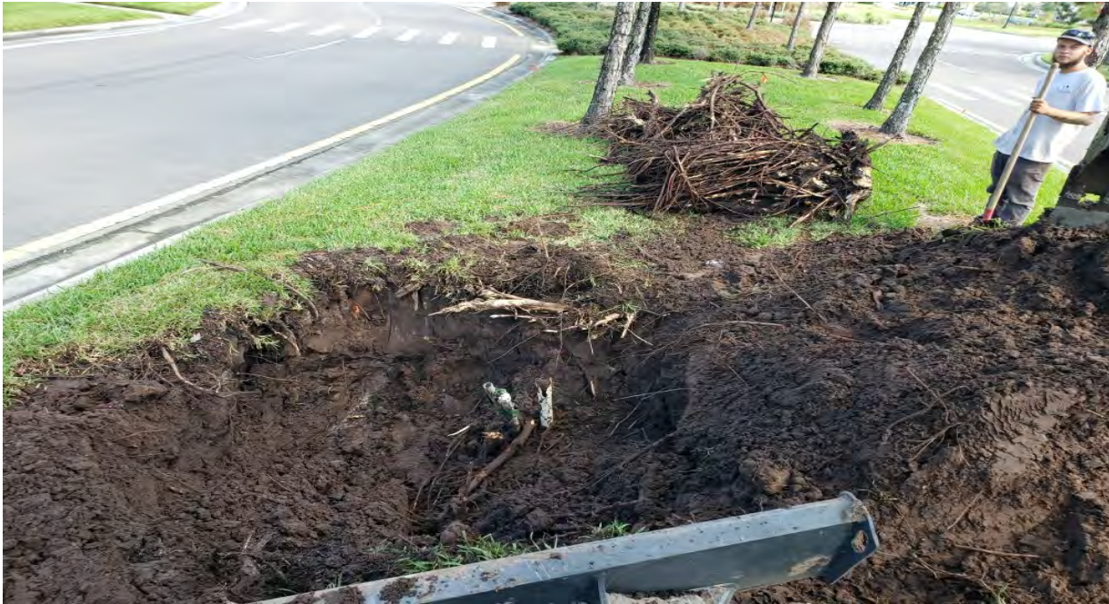
Mainline repair on Connerton Blvd.
